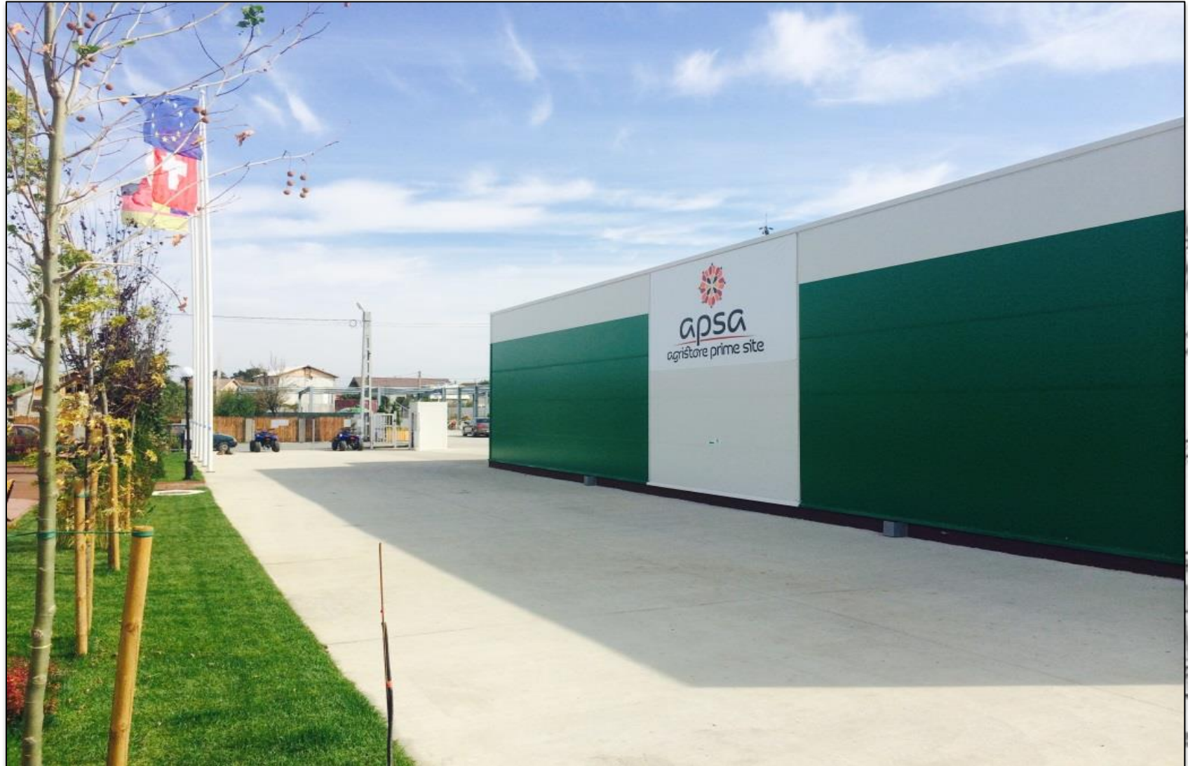
APSA AGRICOSTORE PRIME SITE - MARACINENI (Infrastructure, suprastructure, architecture & facilities)
