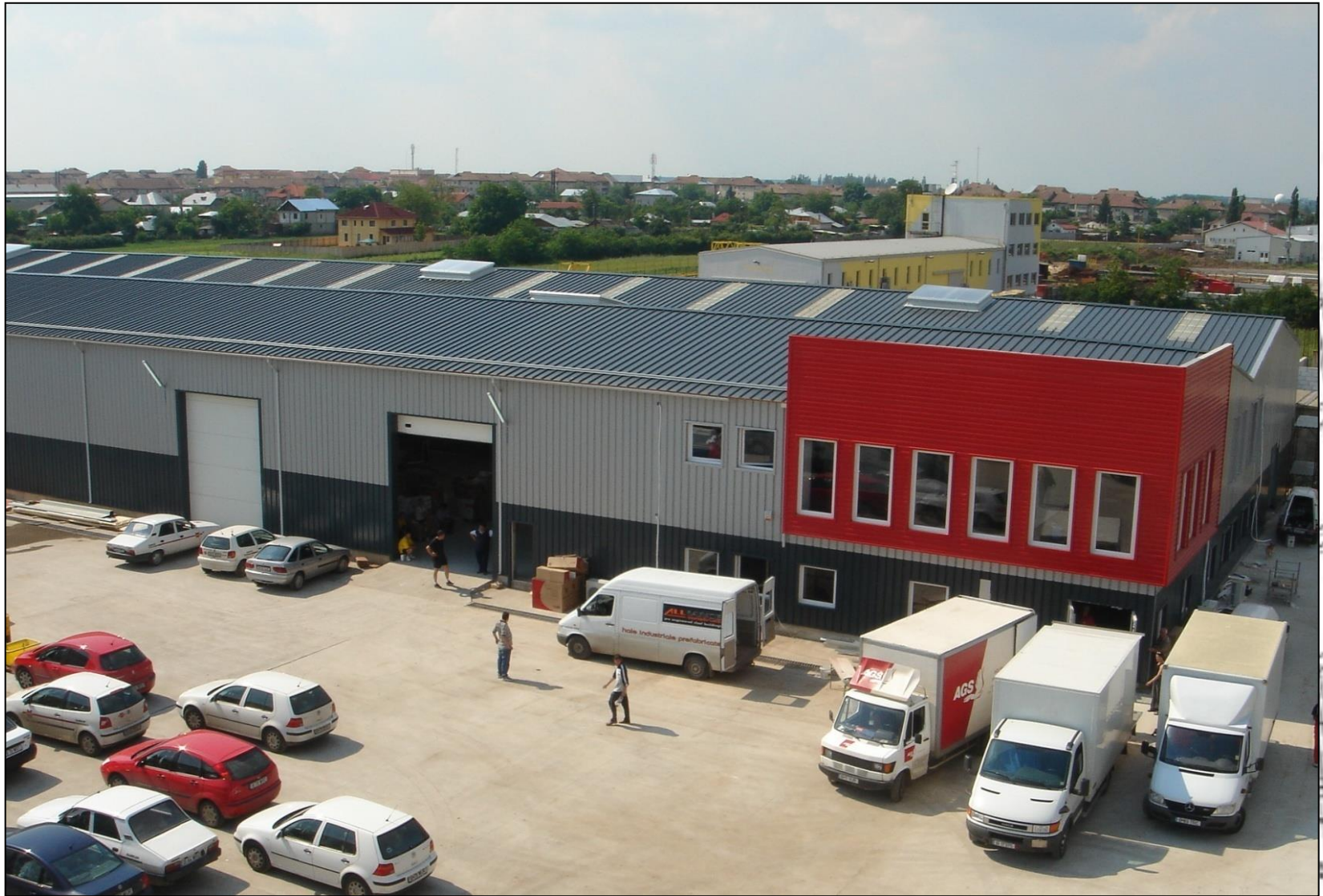
DECA OTOPENI- LOGISTIC CENTER - ( Infrastructure, suprastructure, architecture & facilities)
