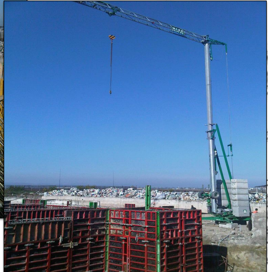
GREENTECH SA – WASTEWATER TREATMENT PLANT ( Infrastructure, suprastructure, architecture & facilities)
