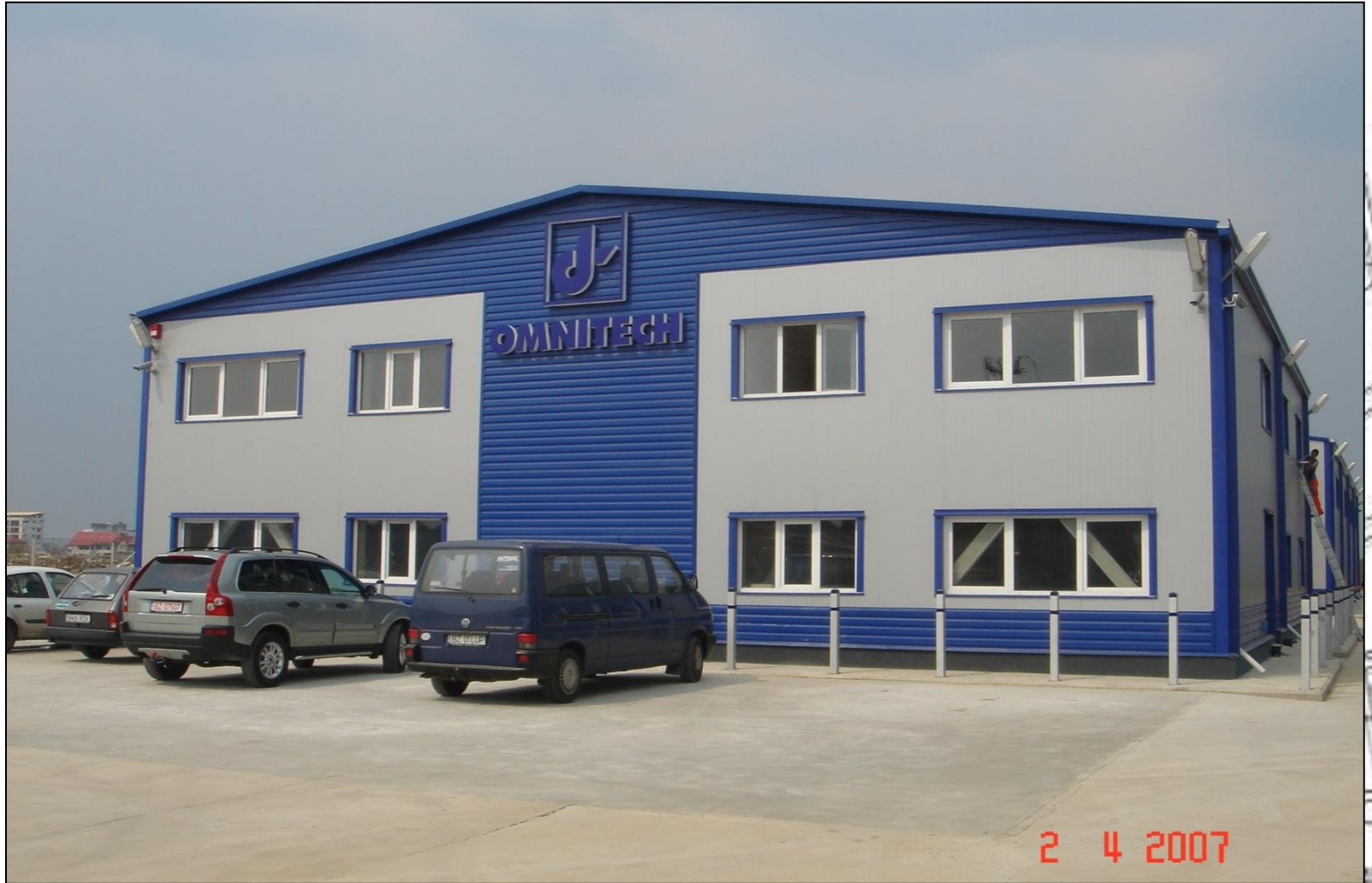
OMNITECH TRADING – OTOPENI ( Infrastructure, suprastructure, architecture & facilities)
