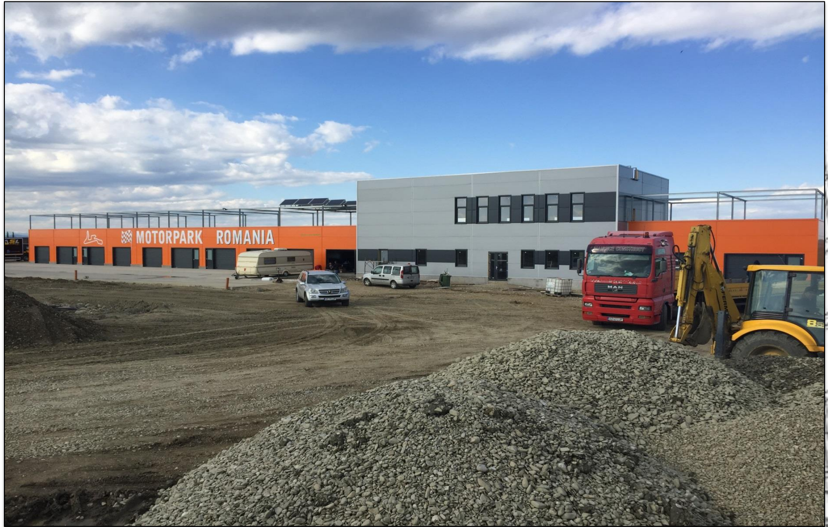
MOTOR PARK – FIRST ROMANIAN FORMULA 1 TRACK ( Infrastructure, suprastructure, architecture & facilities)
