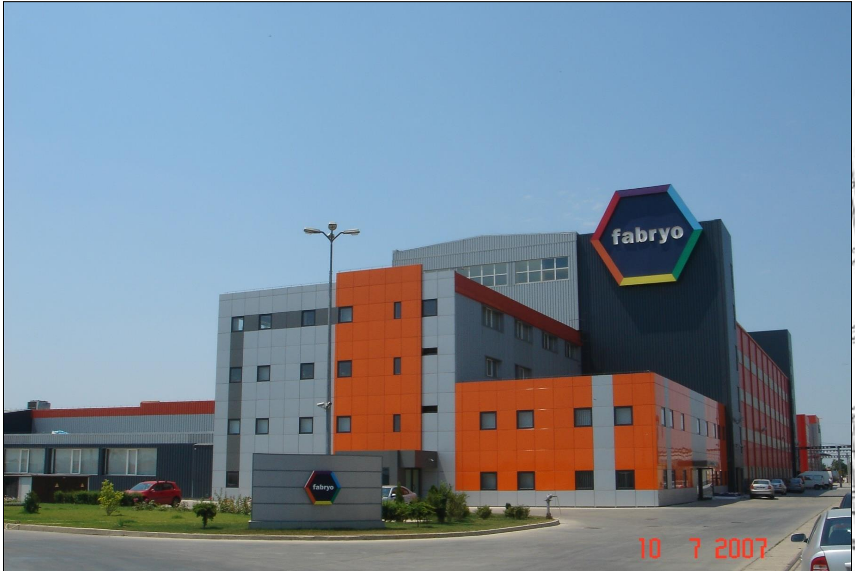
FABRYO CORPORATION - ( Infrastructure, suprastructure, architecture & facilities)
