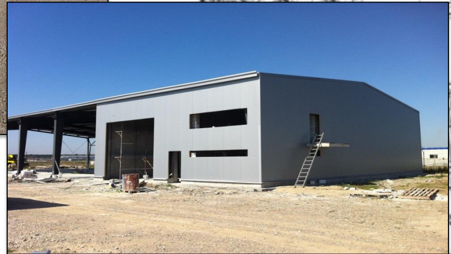
ROMCARBON SA – STEFANESTI ( Infrastructure, suprastructure, architecture & facilities)
