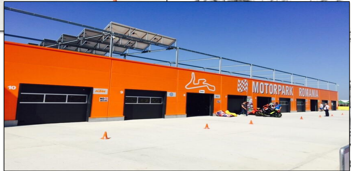
MOTOR PARK – FIRST ROMANIAN FORMULA 1 TRACK ( Infrastructure, suprastructure, architecture & facilities)
